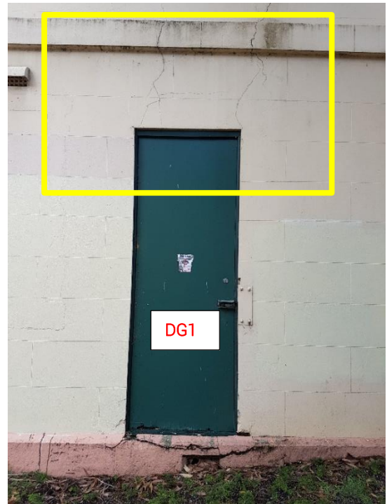
Figure 20 & Figure 21 – South West elevation – lintels to be replaced and surfaces rerendered
