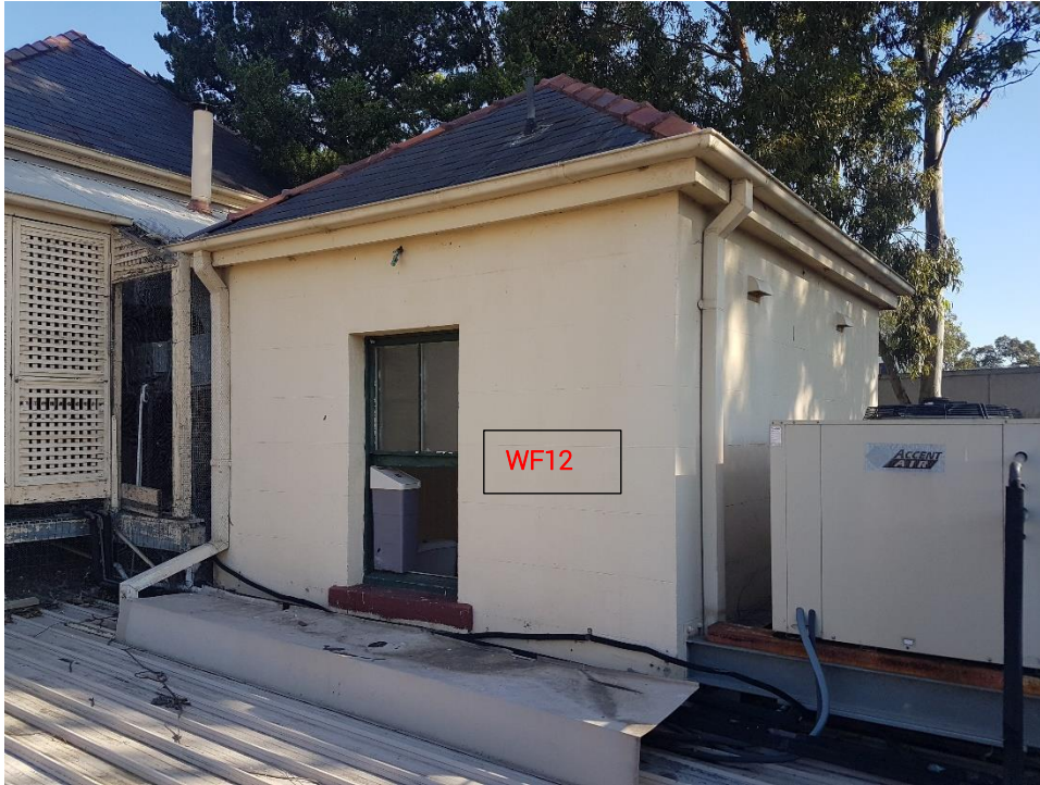
Figure 16 – The Services Building – first floor
