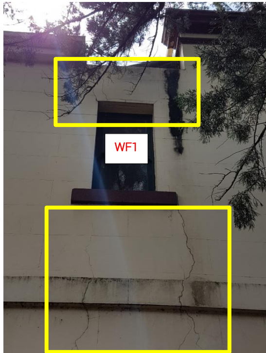
Figure 20 & Figure 21 – South West elevation – lintels to be replaced and surfaces rerendered
