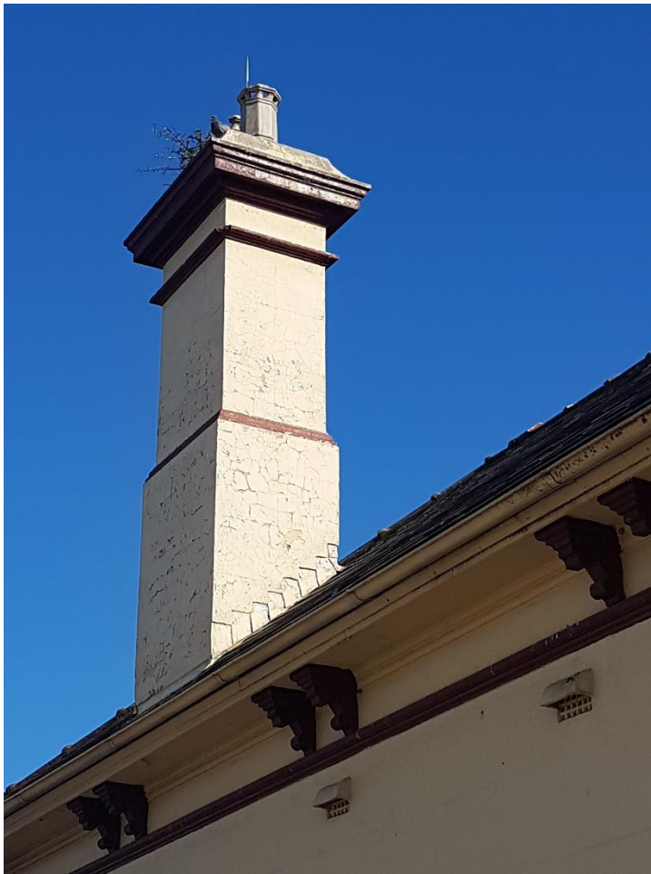
Figure 6 – Chimney Stack 1, North East Elevation, Main Building
