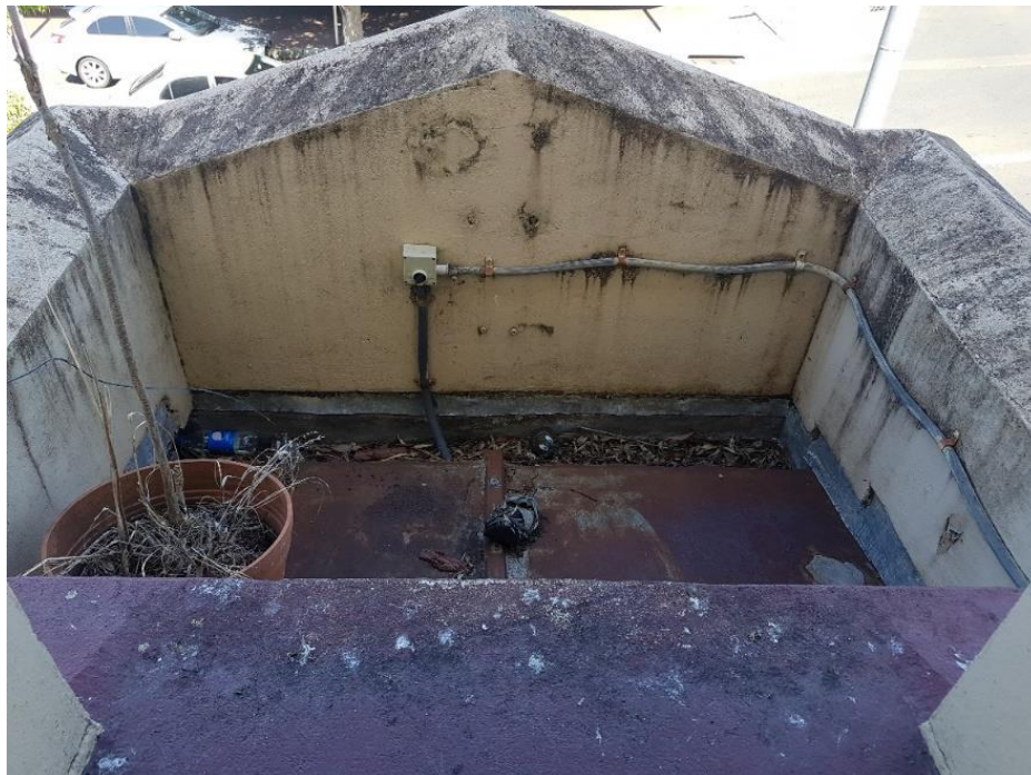
Figure 9 – Roof of the Queen Street porch
