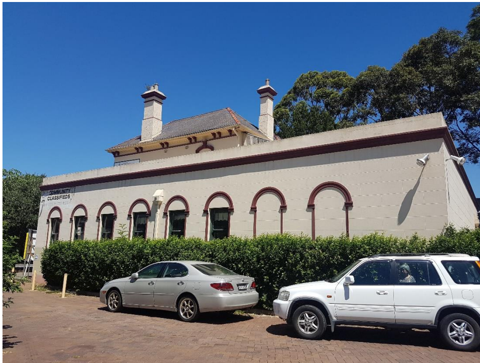
Figure 12 – Single storey building to be demolished
