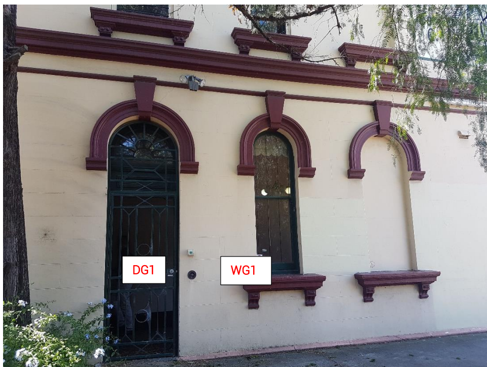
Figure 18 – South West elevation, ground floor - Main Building
