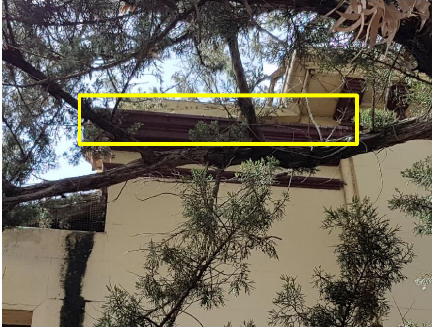
Figure 19 – South West elevation, ground floor - Main Building
