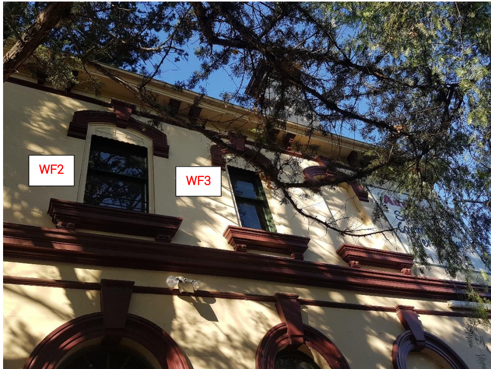
Figure 17 – South West elevation, first floor - Main Building
